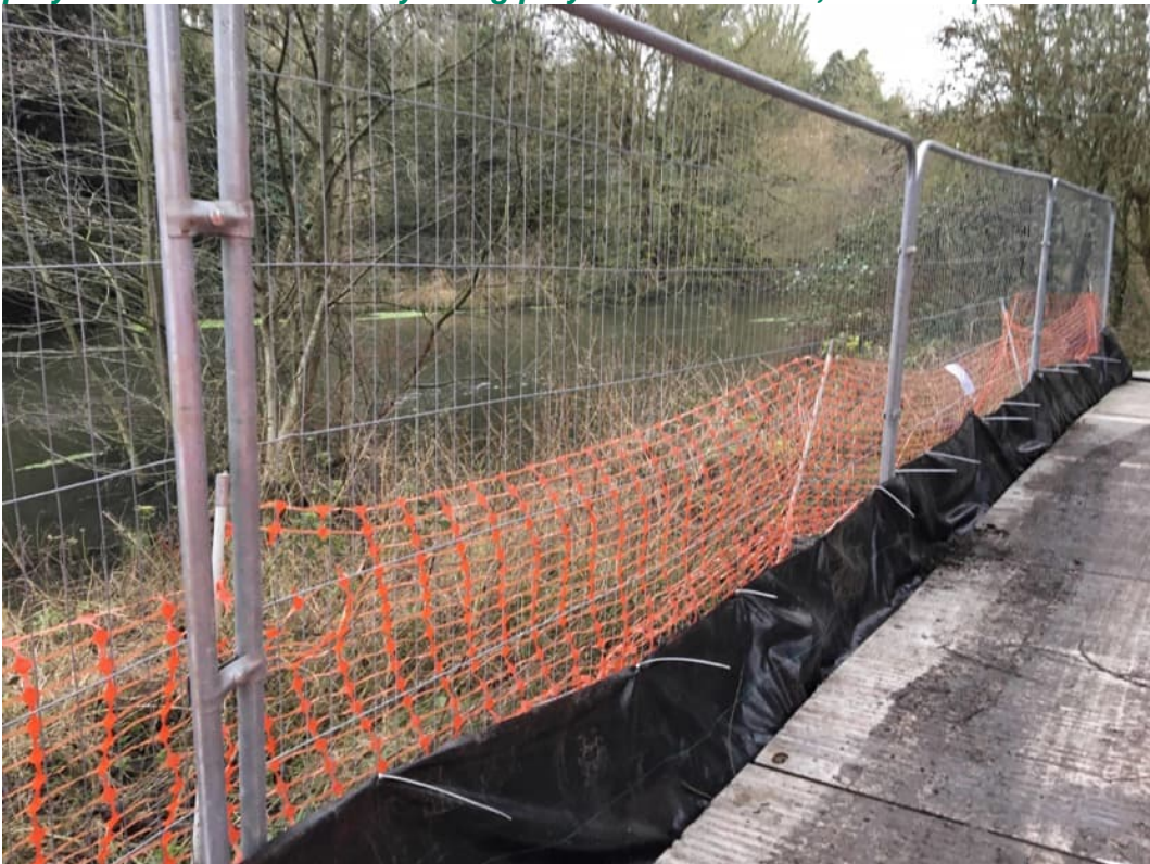
Example of biosecurity fencing adjacent to soil protection (track matting with polythene underlay) polythene collar created by fixing polythene to Herras, for extra protection
